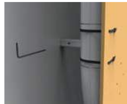
6. Detail of the wall pins fixing.
