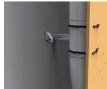
7. Detail of the wall pins fixing.
