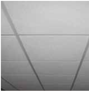
Suspended T-bar & ceiling tiles (min. 8 mm)
